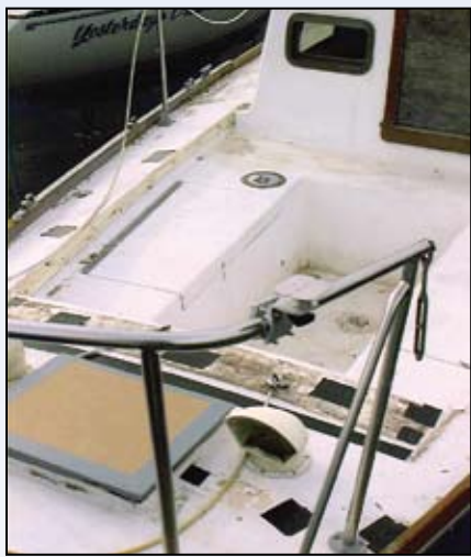
Deck work begins with removal of all hardware.
